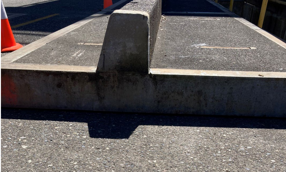
Photo of deck plate on roadway.
